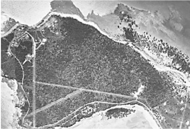
East Point monsoon forest in 1943 during military construction. Photo courtesy of Franklin et al., 2010
